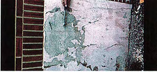
(Delaminated Concrete)
